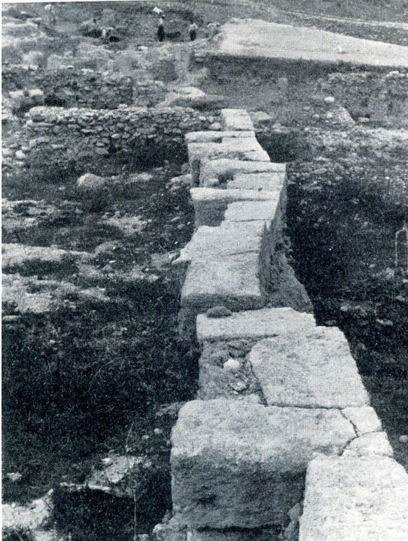
Picture Fig.1: Shifting undergone by the foundations of the façade of a building in Ugarit, collapsed during the earthquake of 1365 BC.
